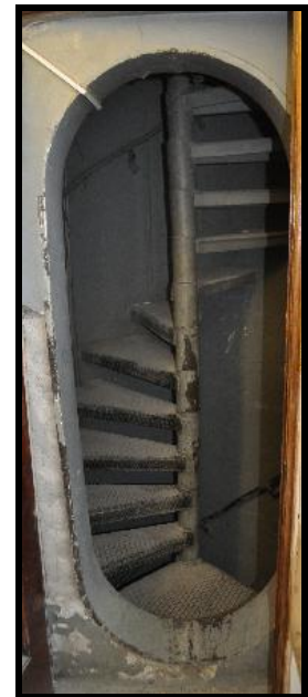
The Secret Stair shaft - 2A22
