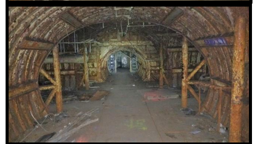
The Lower halls at -3; more rust and erosion
